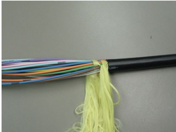
Figure 5: Separate Aramid Yarn
