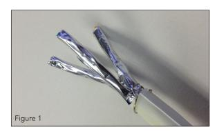
4.2 For 568B wiring, trim foil on orange and brown pairs to ½". Trim foil on blue and green pairs to 1/8". See Figure 2. **Note:** For 568A wiring, trim foil on the green and brown pairs to ½" and the blue and orange pairs to 1/8".
