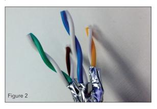
4.3 Orient wire pairs into correct position and according to the color code guide on the jack. housing. See Figure 3.
