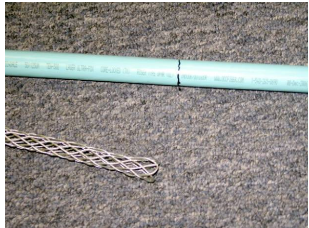
Figure 2: Marking Cable Where Pulling Grip Ends
